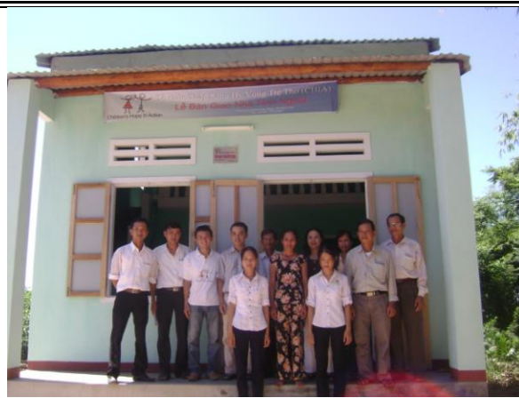
P6. House of Thuy TTT, XXX Commune, XXX District after supported by CHIA
