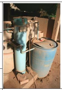
Figure 1 Measuring tank (left), Storage tank (right)
