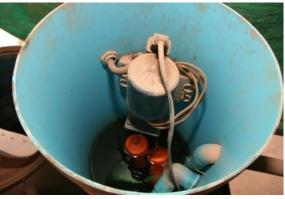
Figure 02 Measuring Tank with Floating Switch Visible
