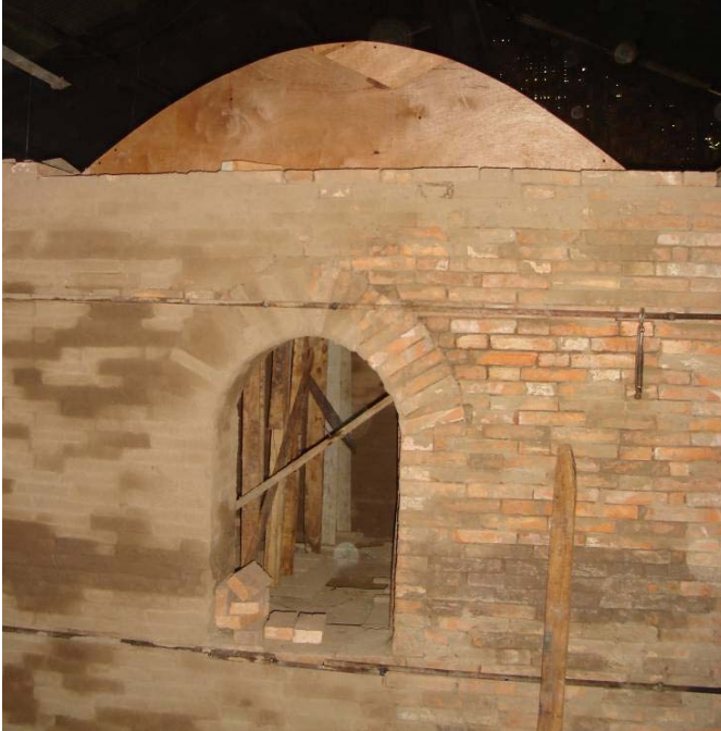
Interior bracing during roof construction.
