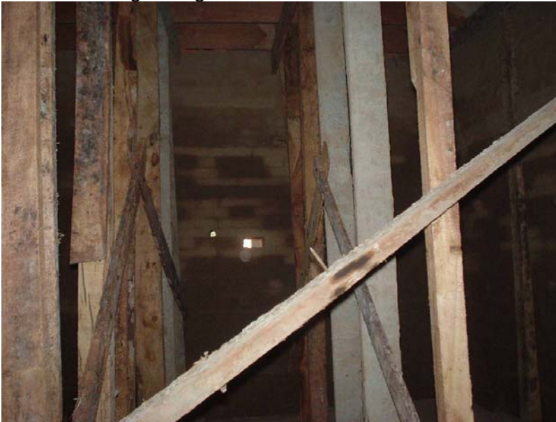
Interior bracing during roof construction.
