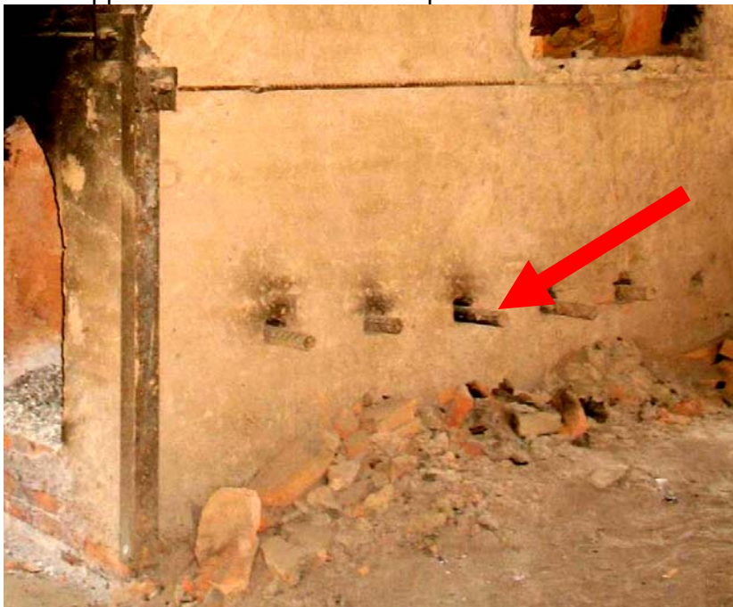
Fuel support rods installed in a completed kiln.
