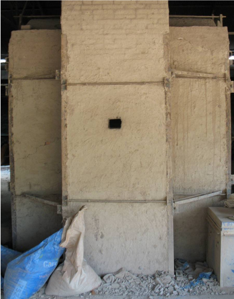
Steel reinforcement of kiln chimney.
