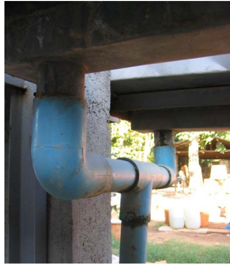
Figure 4.17 Drainage for filter racks
