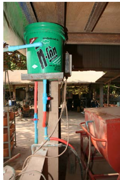
Figure 4.12 Alternative Spray Water System - Raised bucket with adjustable overflow at between 12 and 15L gravity feeds into clay mixer through spray pipe
