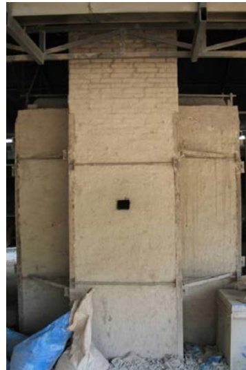
Figure 4.6 Kiln from back - with chimney
