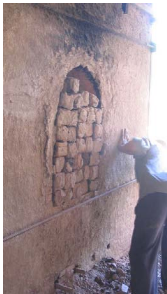
Figure 4.10 Worker closing kiln opening tightly with bricks
